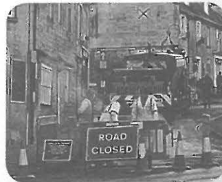
5 Repairs to streets and freeways. (4, 4)
